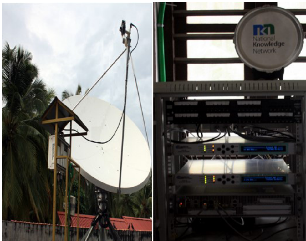
Figure 4 : High Capacity SCPC VSAT at Kavaratti, the U.T. of Lakshadweep Island for NKN Project
